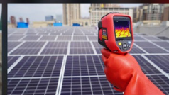
Photovoltaic Panels Inspection
