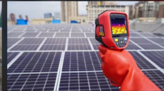
Photovoltaic Panels Inspection
